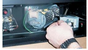
5. Attach the yellow terminal connectors to terminals on the blower. Be careful not to break the terminals off the blower.
