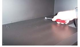
Locate the two mounting tabs in the rear of the valve chamber. Bend both tabs up <u>90 degrees.</u>
