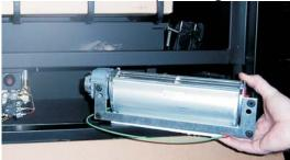
3. Place the blower on it's back and slide it into the valve chamber. Be very careful not to bump the electrical terminals, they are very fragile.
