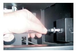
15. Plug the blower power cord into the receptacle. Restore the power to the fireplace.
